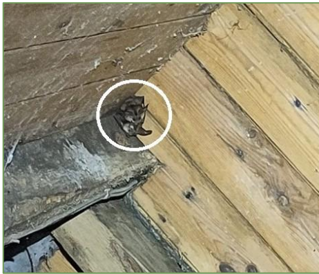
Plate 3.3 –Brown Long-eared Bats roosting in S02 on internal inspection.
